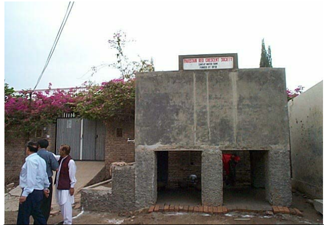
Water tank installed by the PRCS in Jughian village, Punjab Province.
