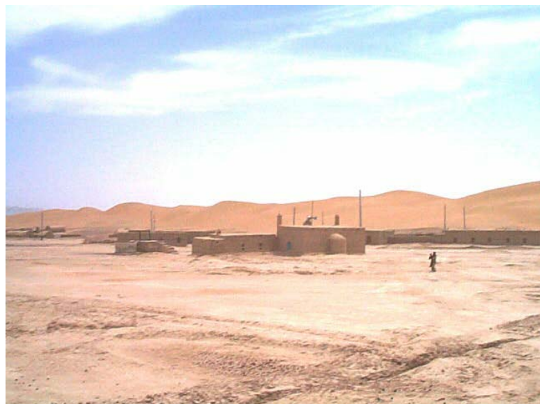
Disater Mitigation Project Site in Baluchistan Province
