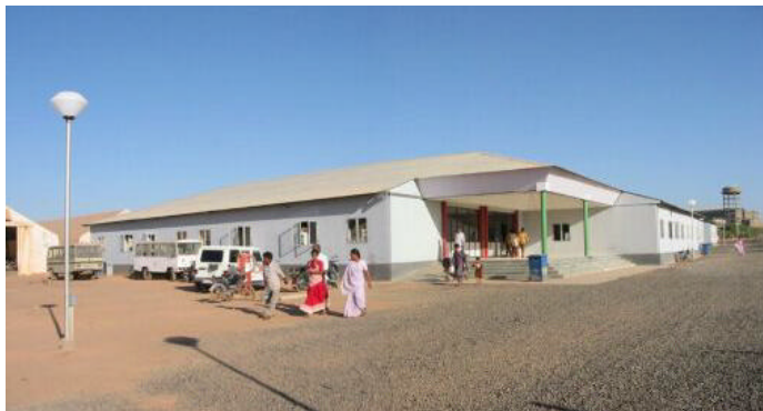
After seven months of construction, the 204-bed general hospital on the same site as the ECHO funded emergency referral hospital in Bhuj was handed over to the health authority of Gujarat.
