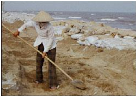
Mrs Nguyen Thi Ngoc is repairing a broken sea dyke in Hai Thinh.
