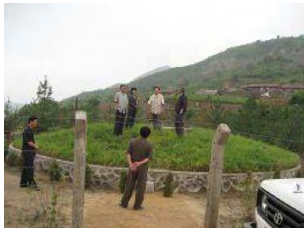
Newly constructed storage tank in Songjong ri, Hamju County, South Hamgyong province. DPRK RCS.
