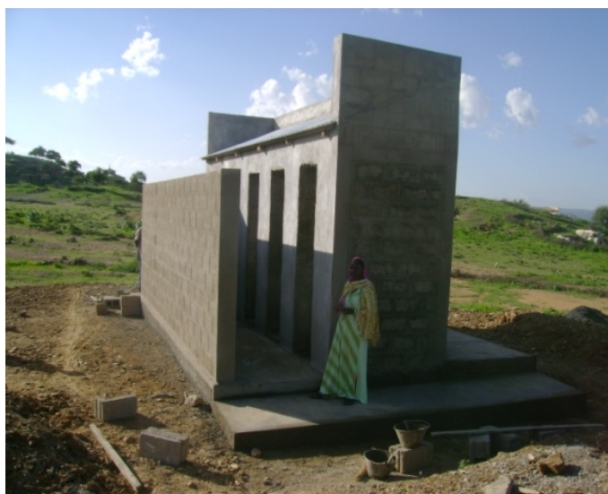
Tserona school latrine, August 2009
