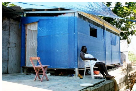
After the devastating earthquake on 12 January 2010, the Red Cross Red Crescent National Societies provided shelter support to the affected population. The picture shows a transitional shelter built by the Spanish Red Cross in Leogane, Haiti. IFRC
