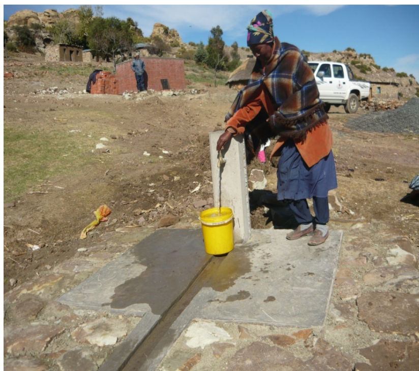
A community member filling a water bucket from a newly constructed water point in Mafeteng District. Photo: Lesotho Red Cross
