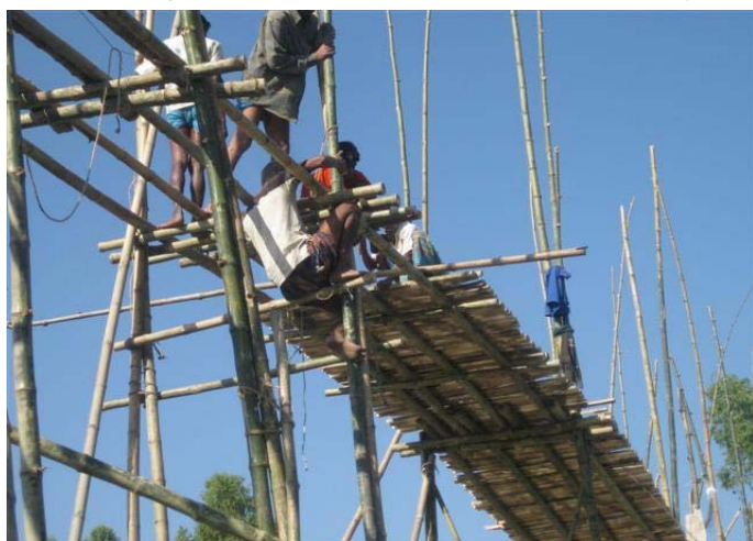
A bamboo bridge constructed by the community under the CBDRR project. Photo: IFRC
