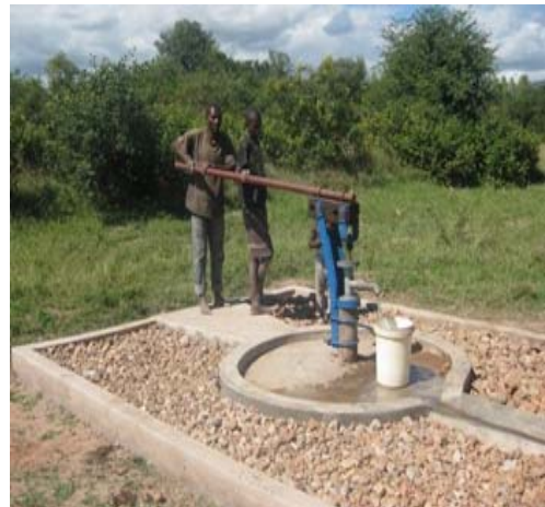
Rehabilitated borehole in Mutare District, Manicaland
