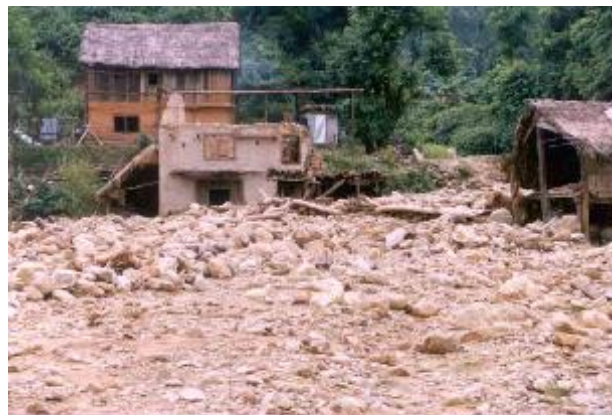
Landslide damaged a home of Jyamsire WRL, Mahottari in Makwanpur district.
