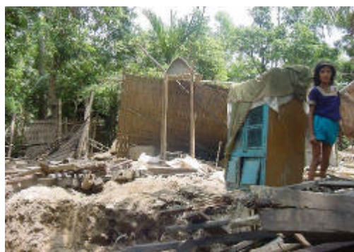
Damage house affected by flash floods at Feni
