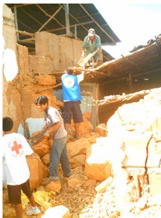
Red Cross Volunteers removing rubble from destroyed houses in Moyobamba.
