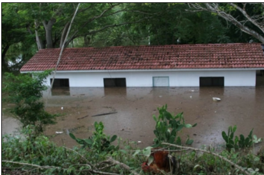
Flooded house in the affected states in Mexico. Source: Mexican Red Cross
