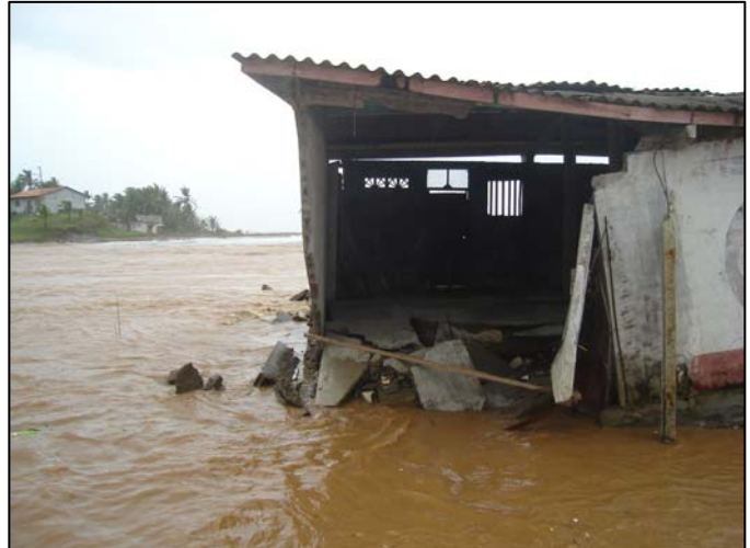
Overflowing of the rivers caused severe flooding Source: International Federation.
