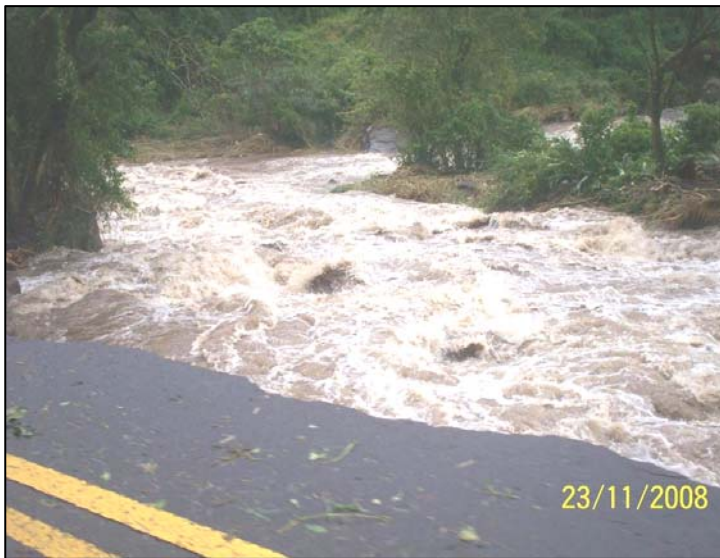
Overflowed river destroyed a road in Chiriqui.
