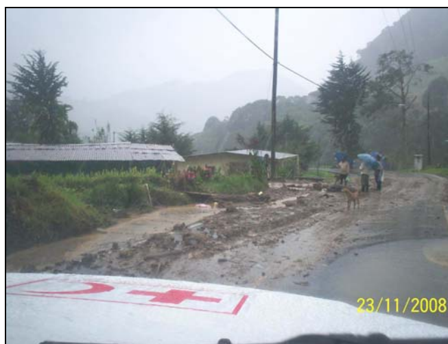
The roads in the province of Chiriqui were severely damaged by the heavy rainfall. Source: Red Cross Society of Panama.
