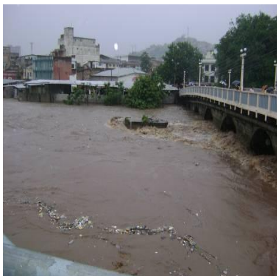
Floods in Tegucigalpa Source: Honduran Red Cross Society
