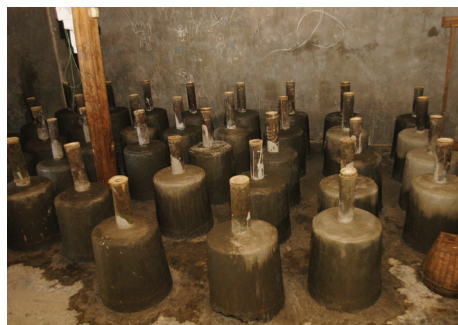
Foundation pads cast with bamboo to connect them to the frame
