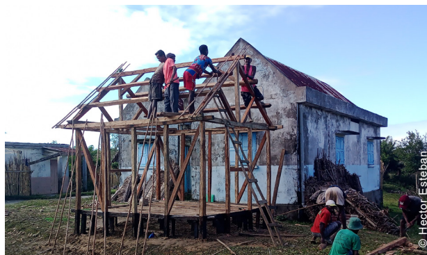
Building of a model house with trained carpenters, Conditional Cash for Shelter program.
