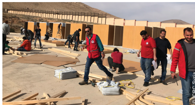
Works were implemented by contractors, who then were also hired for the maintenance phase.
