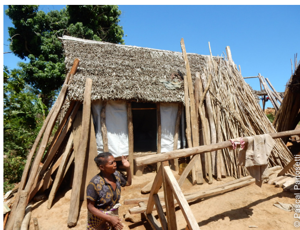
House repairing process with Conditional Cash for Shelter approach.
