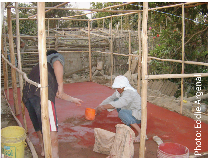
Making the concrete floor slab
