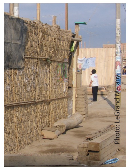
One of the project's shelters (background) and a shelter walled with reed mats (foreground)
