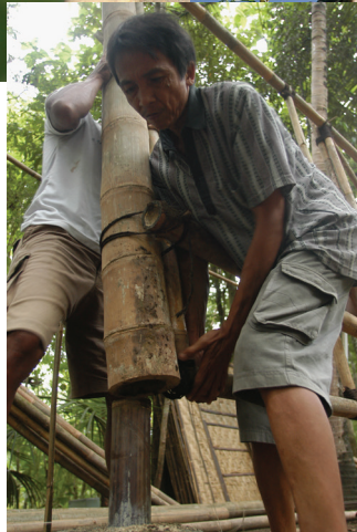
Connecting a vertical post to the foundation
