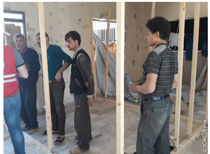
Shelter kits were used to build indoor partitions to increase privacy.
