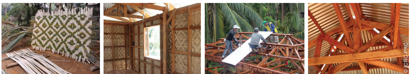
The project used locally available materials (e.g. the amakan sheet, left) and safe construction techniques, including bracing, strong trusses and roof strapping.
