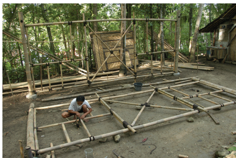
Prefabrication of a wall panel
